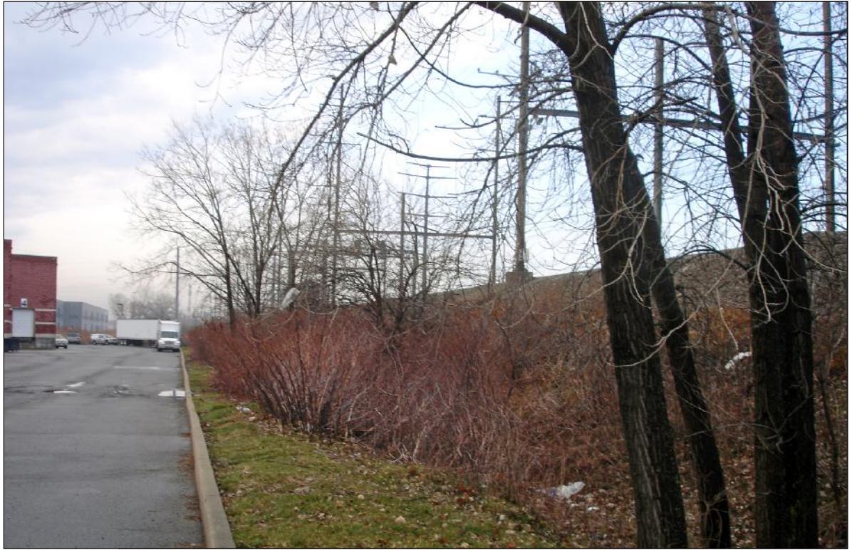
NEC embankment at 901 Penhorn Avenue Parking lot/loading docks, facing west 1
