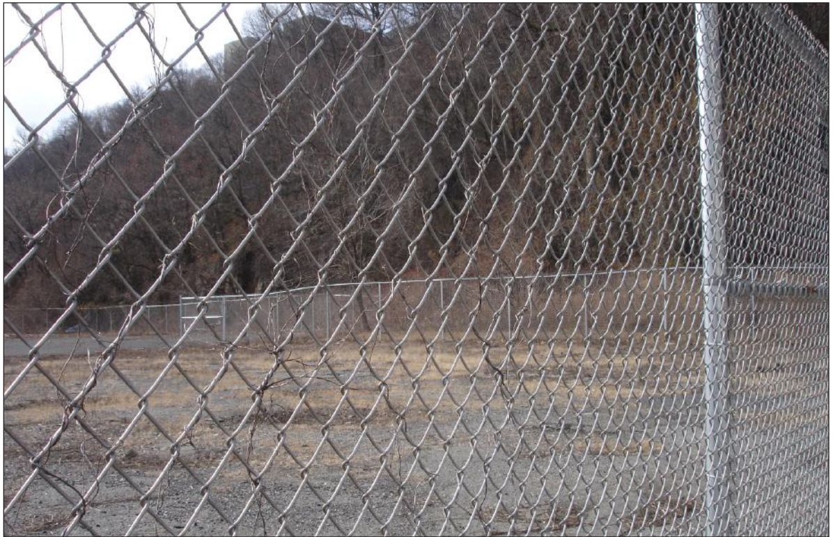
Hoboken fan plant site from West 18th Street in Weehawken, facing west 8
